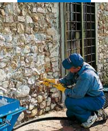
Consolidating injection with Mape-Antique I
