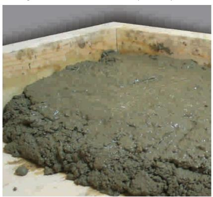
2. Base Concrete or Lime Mortar Pour ½ depth of concrete or lime mortar Work mixture to eliminate any air pockets
