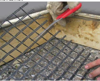
1. Measure and Cut Extend grid to 2.5-5.0 cm of forms. Overlap seams by 2.5-5.0 cm
