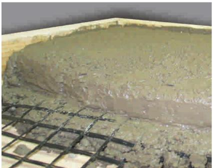
4. Finish concrete or lime mortarComplete concrete or lime mortar pouring and surface finishUser is responsible for product selection, handling and application.
