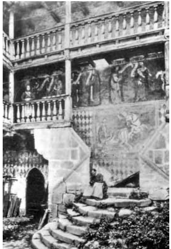
Figure 302. Castle of Fénis, Piedmont: courtyard before restoration (prior 1897). This castle served as a model for the 'Borgo' in 1884
