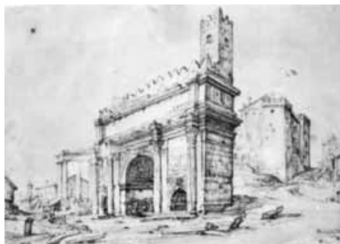
Figure 12. The Arch of Septimius Severus, Rome, with remains of mediaeval structures (M. Brill)
