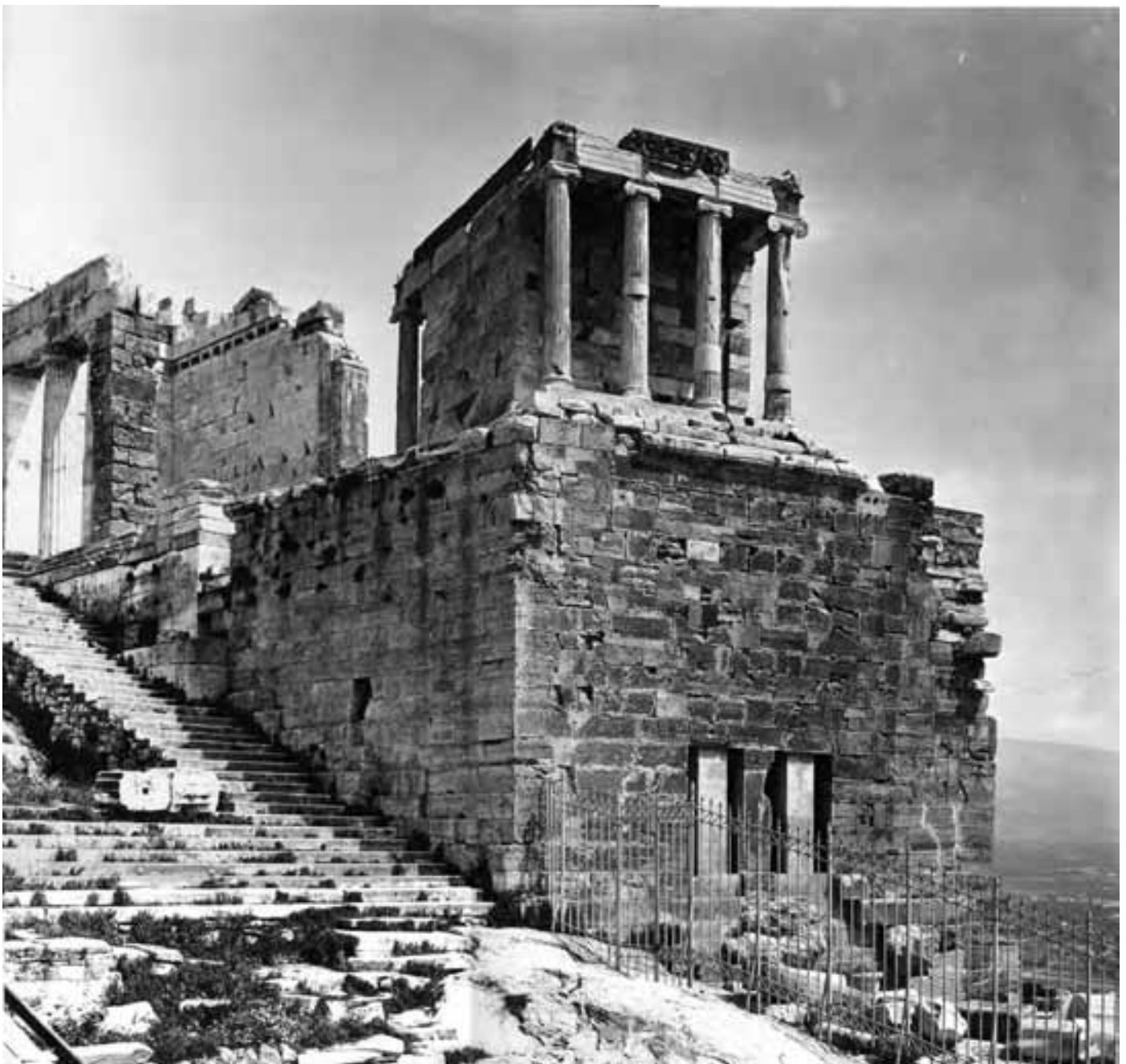
Figure 125. The Temple of Athena Nike c. 1900. The basreliefs have been replaced with terracotta copies from the originals in the British Museum (Elgin Marbles); losses have been integrated in simple forms with no details
