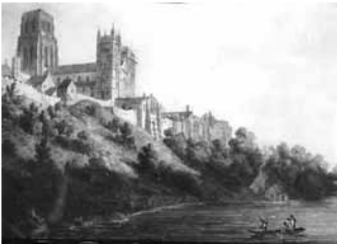
Figure 140. Durham Cathedral. Detail of watercolour by E. Dayes in 1795, showing the scaffolding for the construction of the pinnacles
