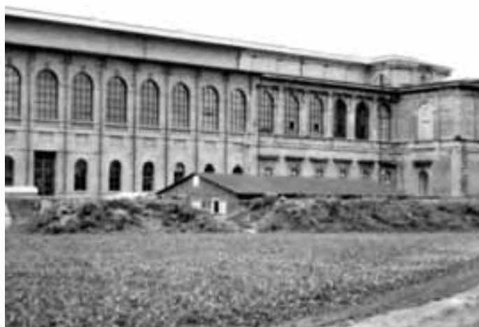
Figure 335. The Pinakothek, Munich, restored after the Second World, respecting historic material
