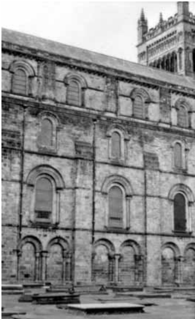
Figure 165. Durham Cathedral, north elevation after restoration
