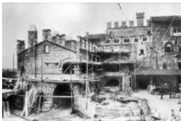
Figure 305. Castle of Pavone during restoration (1893)
