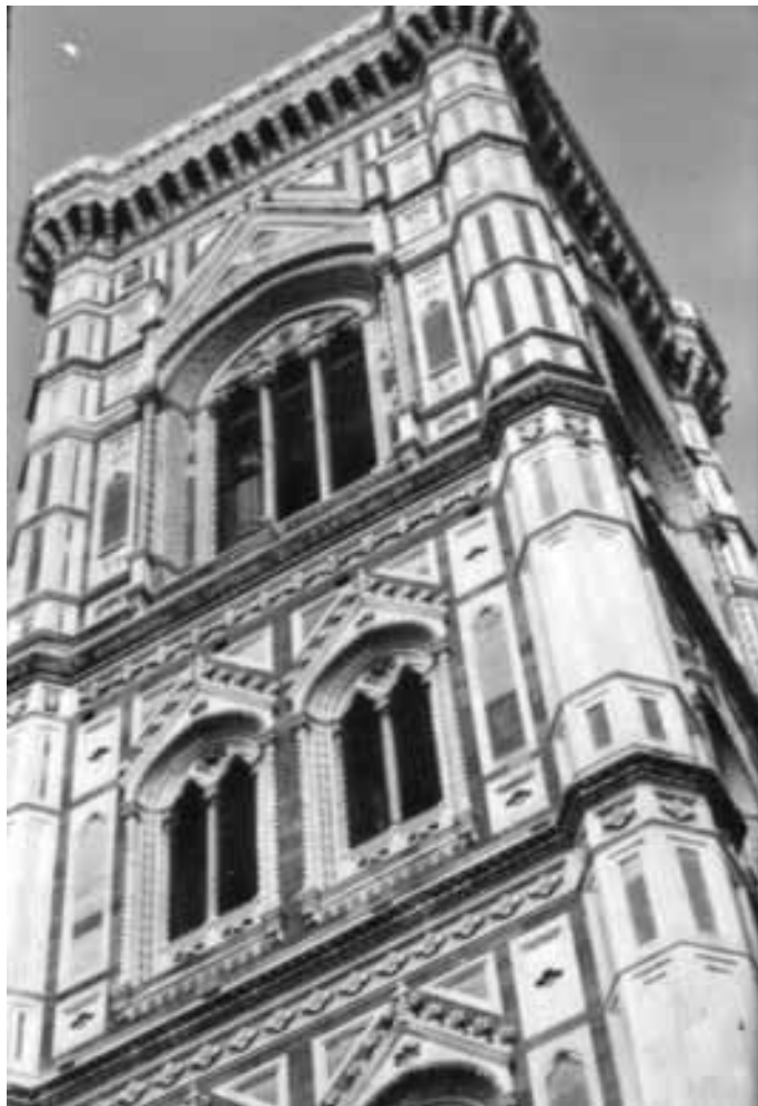
Figure 287. Detail of Giotto's Bell Tower in Florence
