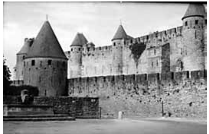
Figure 260. Carcassonne, Le Cité after restoration, photo in 1980
