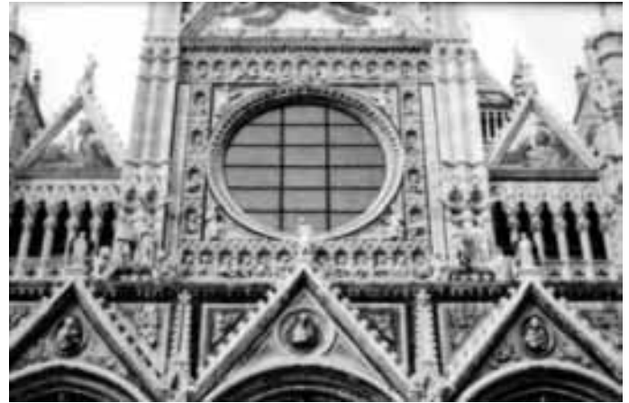
Figure 296. Siena Cathedral, west front after restoration
