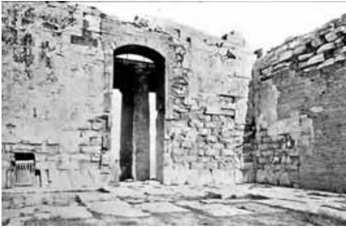
Figure 131. The Parthenon, the interior of the cella c. 1900, showing the 19th-century restoration in brick
