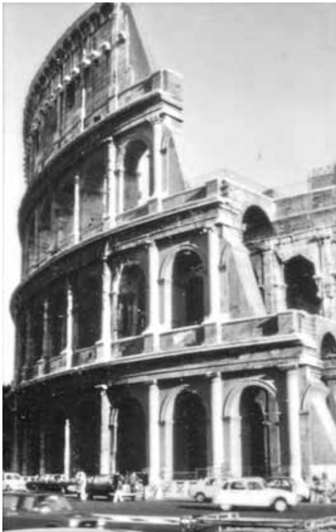
Figure 113. The Colosseum after the construction of the buttress by Valadier for the consolidation of the west wall
