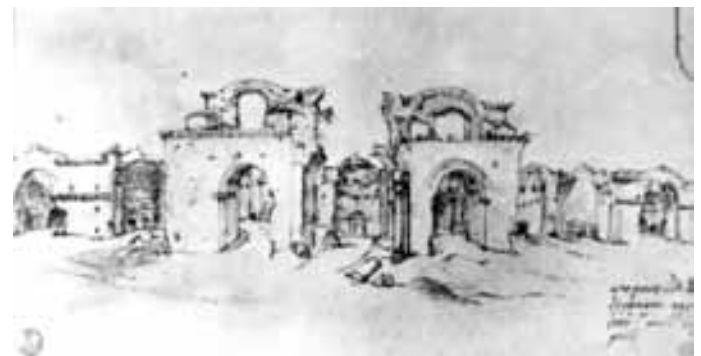
Figure 38. The entrance to the Thermae of Diocletian, Rome, where Michaelangelo built the church of S. Maria degli Angeli
