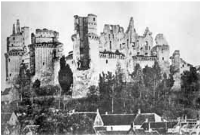
Figure 262. The Castle of Pierrefonds before restoration
