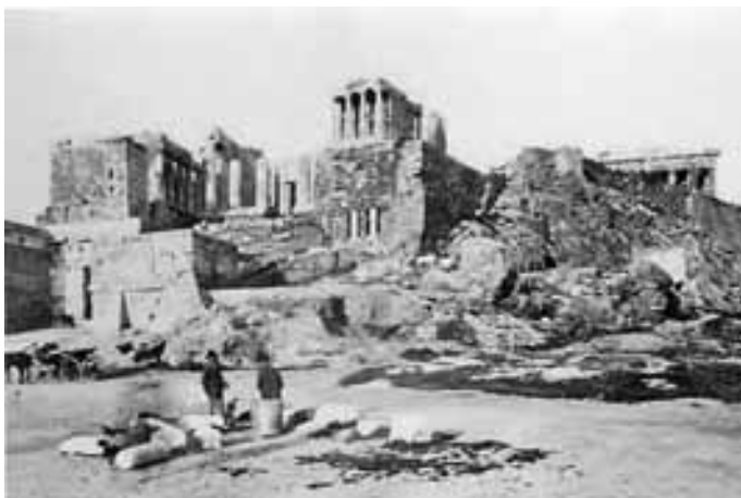
Figure 132. The Acropolis (c. 1900) before the 20th-century restoration works
