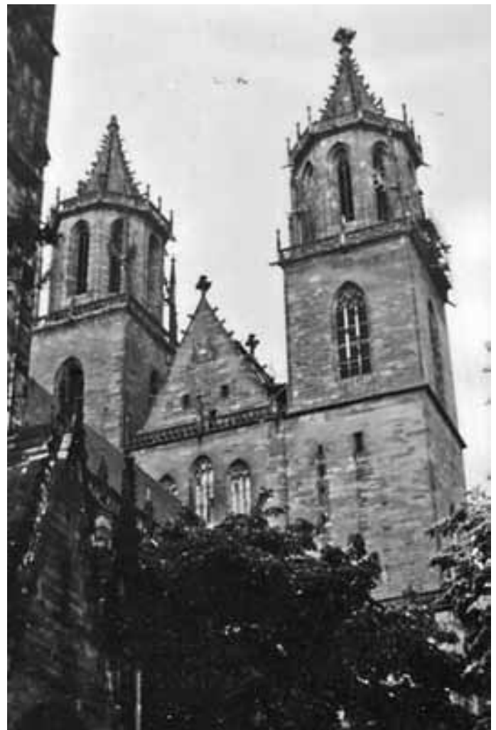
Figure 186. Magdeburg Cathedral, western towers in 1979
