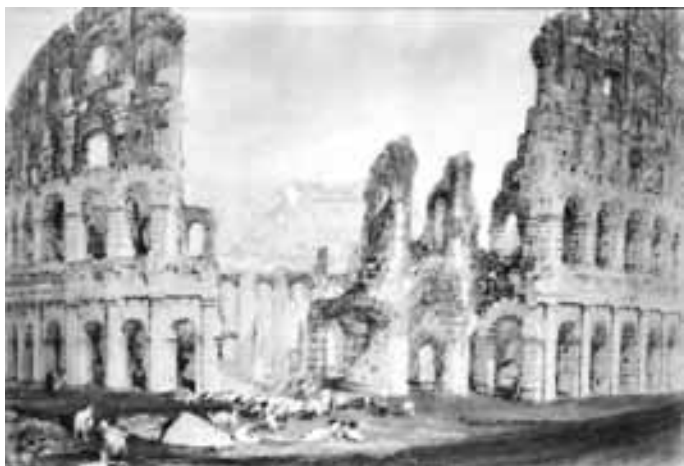
Figure 114. The Colosseum: south wall before restoration (Turner)
