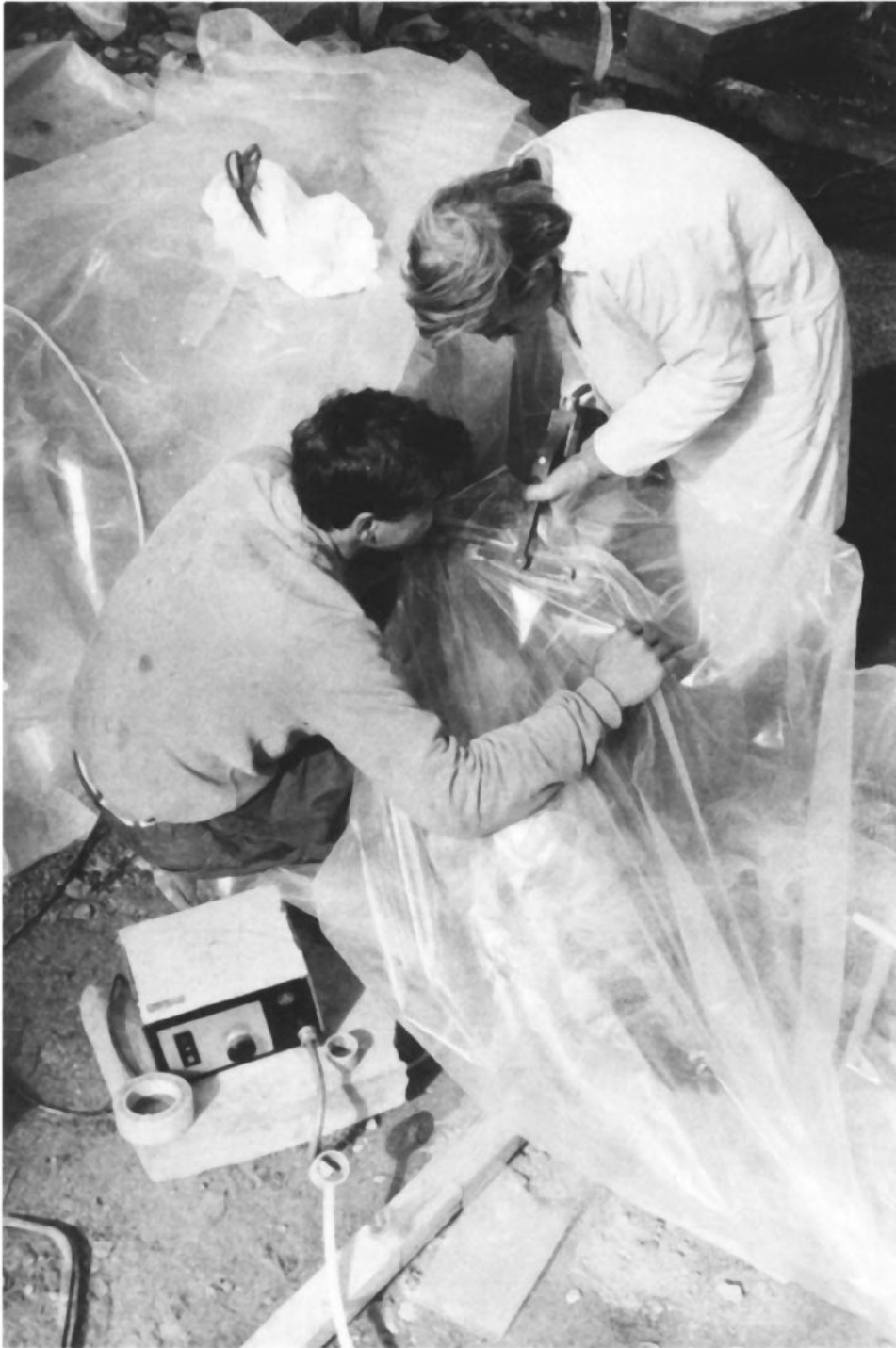
Professor Petr Kotlik (right) and his assistant are heat-sealing polyethylene film to create a containment chamber around a limestone statue as part of a routine program for treating statuary with epoxy resins in solutions.
