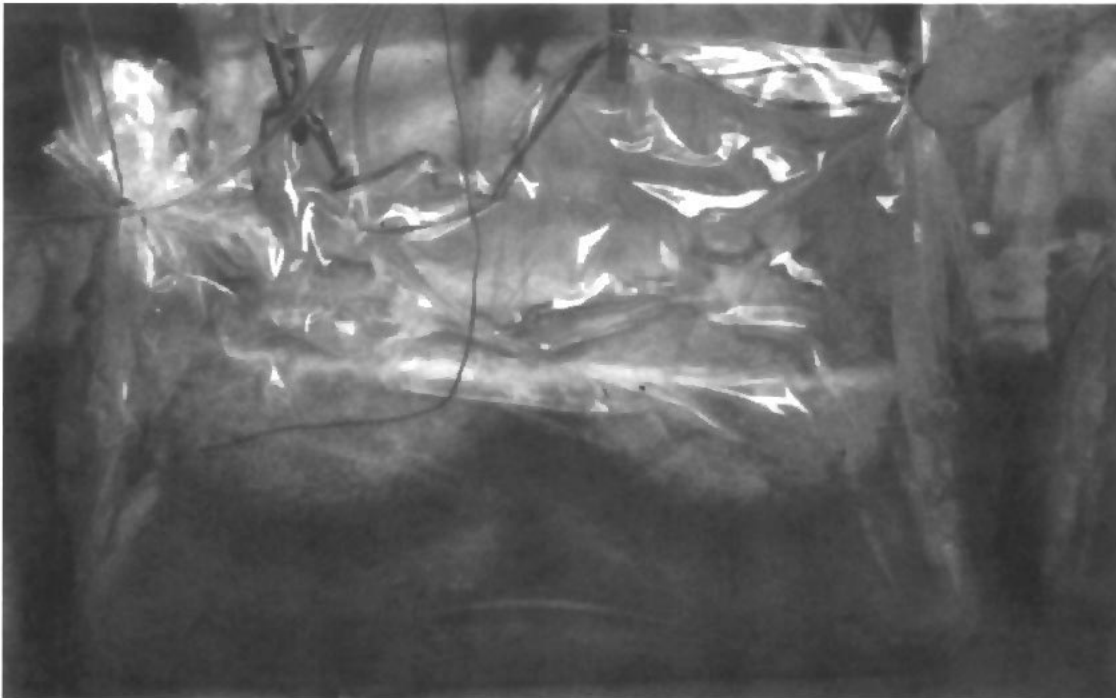
Figure 23. Twin bases of the Basilica of San Andrea treated with resin (Lazzarini 1991).
