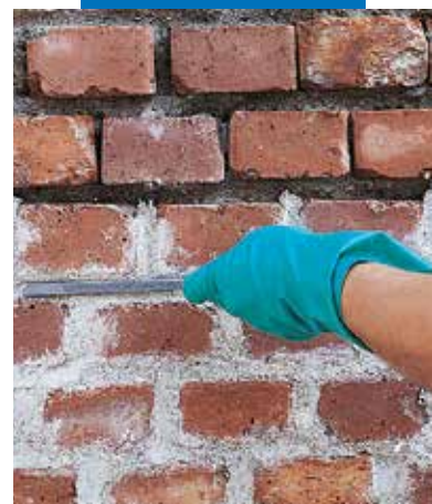
Finishing mortared joints pointed with Mape-Antique MC
