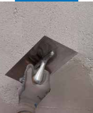
Application of Mape-Antique FC Civile
