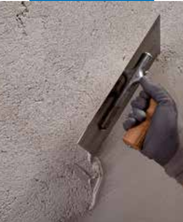
Application of Mape-Antique FC Civile
