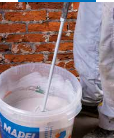
Preparation of Mape-Antique Rinzafo
