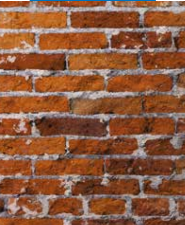
Brick wall after removing the deteriorated render
