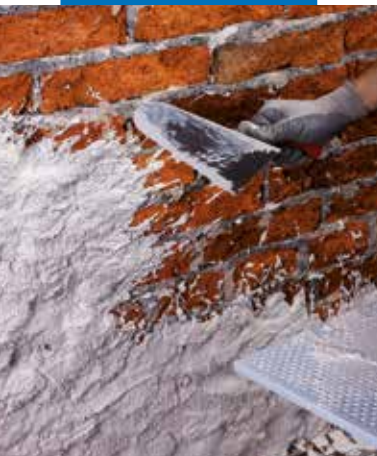
Application of Mape-Antique Rinzafo
