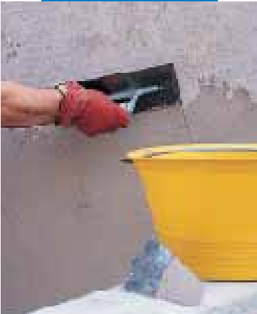
Applying Mape-Antique FC with a trowel
