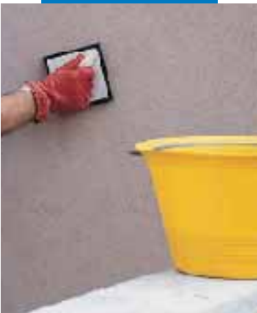
Finishing Mape-Antique FC with a float sponge
